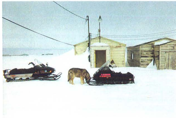
Fig. 2. Top: The variation building that houses the fluxgate magnetometer. Bottom: The main building that contains data collection electronics.
