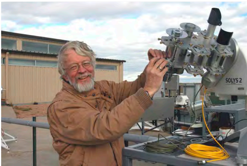
Ells Dutton at the National Renewable Energy Laboratory in 2008 installing pyrheliometers for a year-long comparison of commercial instruments used for direct solar beam measurements.
