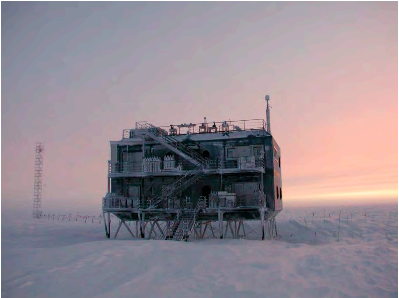
South Pole Observatory
