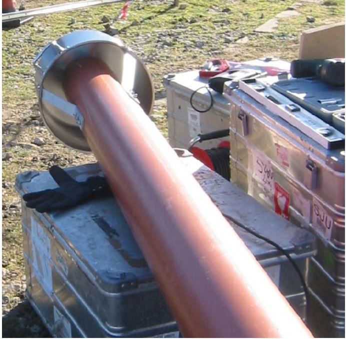
Rain hat connected to top of stack
