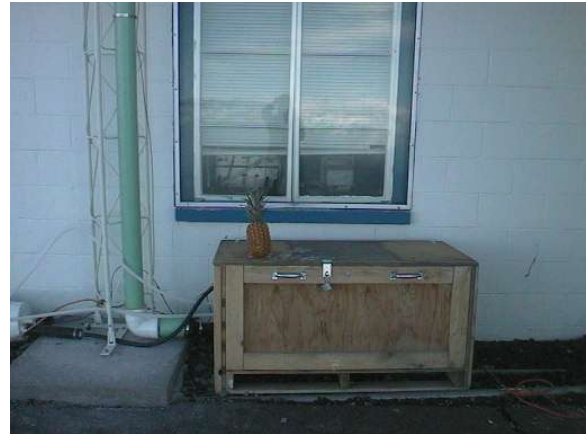
Figure 2-3: Pumpbox at Mauna Loa Observatory. The base of the 10-meter tower and the 10-cm stack bypass line are also seen in the photograph.
