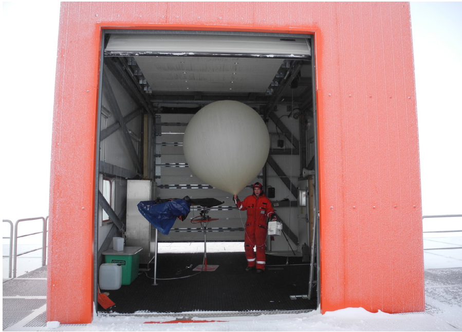
Photo 3: The balloon launching hall located on the roof of the Neumayer III building. Copyright Kathrin Höppner.
