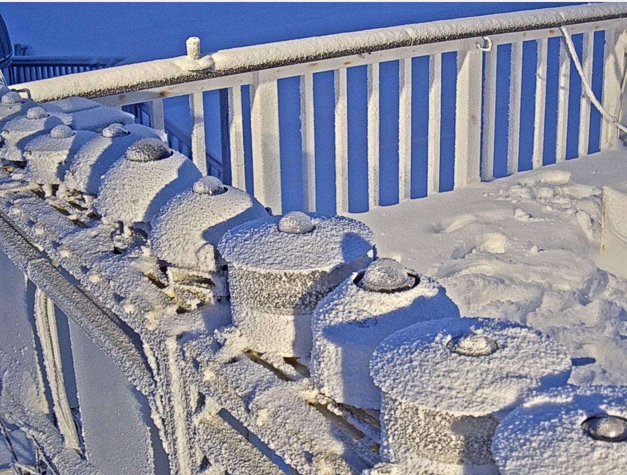
Ventilators Turned Off
